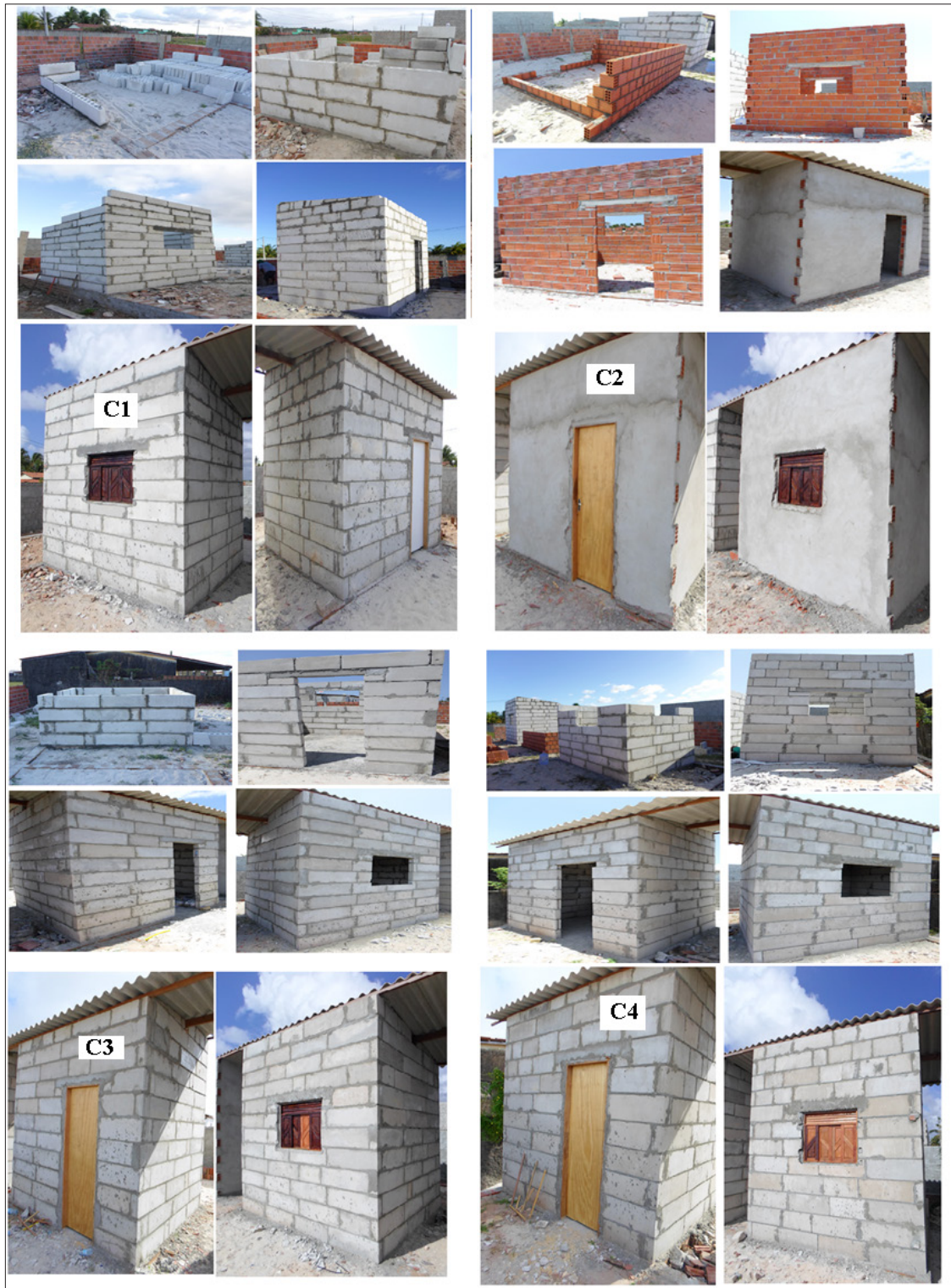
Figure 2: The four rooms under construction and after construction.
